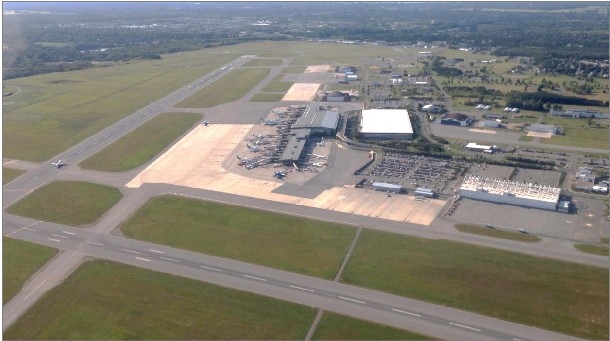
An aerial perspective of the passenger terminal building and surrounding core area at Ottawa International Airport.
